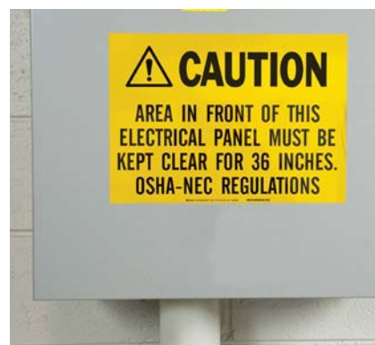
Hazard warning signs
